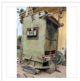
Vertical HT Motor Repairing And Services
